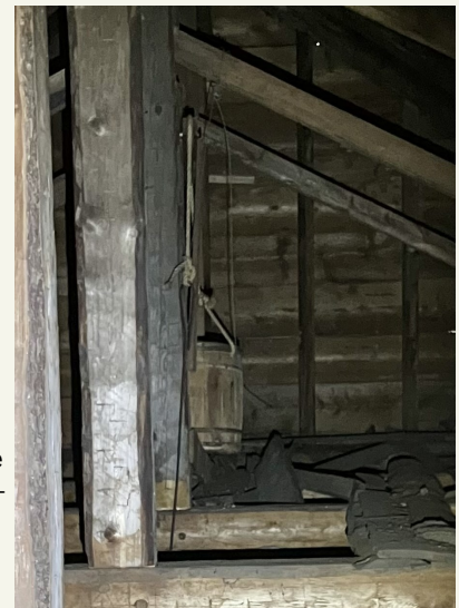
Pulley and bucket counterweight mechanism in the Meeting House.
