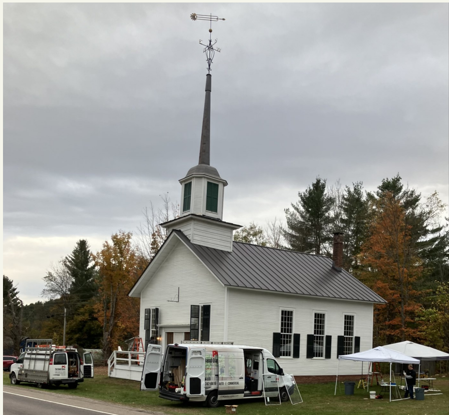
Storm window installation.
