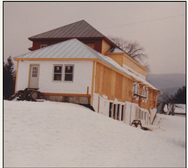
More photos of construction in progress.
