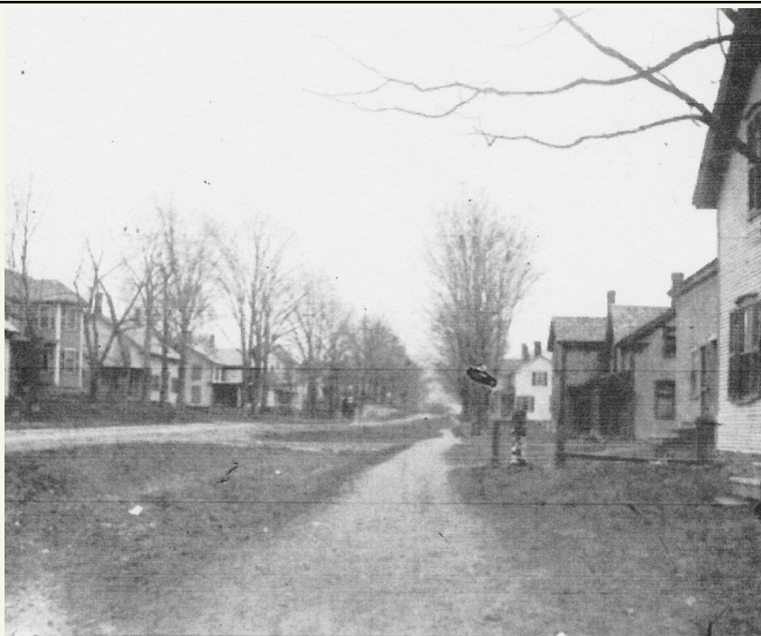
Allen's Garage just visible on the far left of the photograph. Notice the unusual front to the house next to Allen's Garage. This was the Averill home referenced in the newspaper articles.
