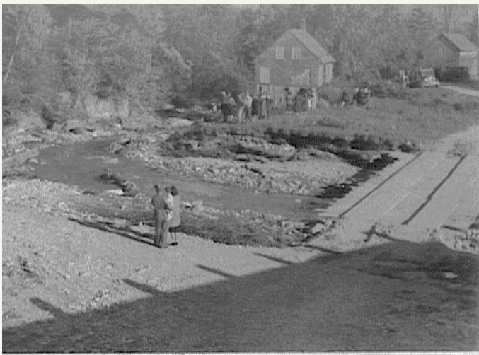
Washed out bridge at Dowsville with temporary bridge installed.
